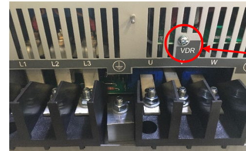
Bottom Terminal Area
